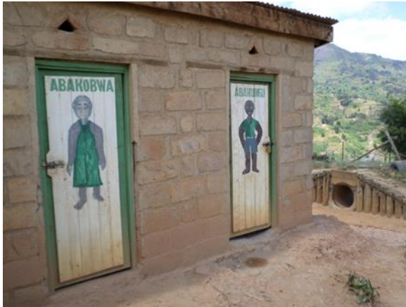
Figure 8. Children's latrines in Kiziba Camp
